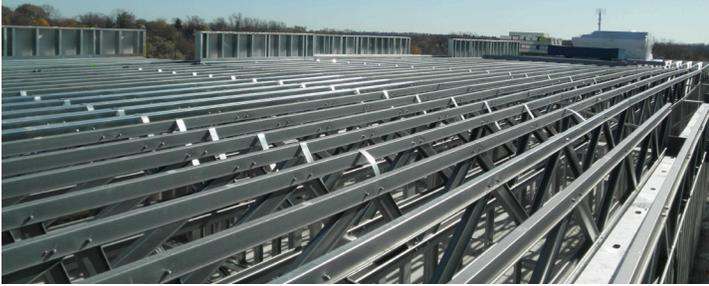
The cold-formed steel roof trusses had a slight slope designed to save money on the project.
