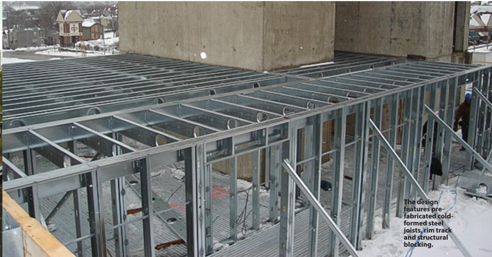
The design features pre-fabricated cold-formed steel joists, rim track and structural blocking.
