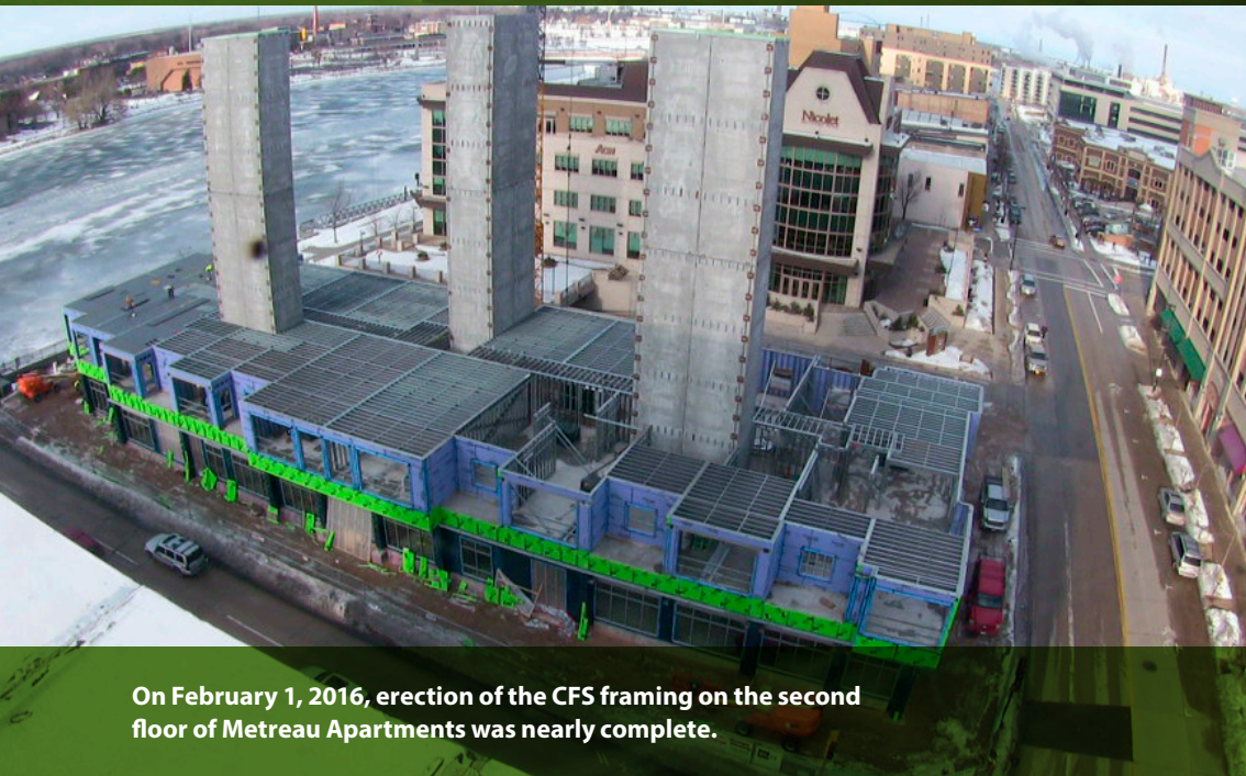
Metreau Apartments' lateral-resisting system includes X-braced CFS shear walls and pre-cast concrete stairs and elevator shafts.
