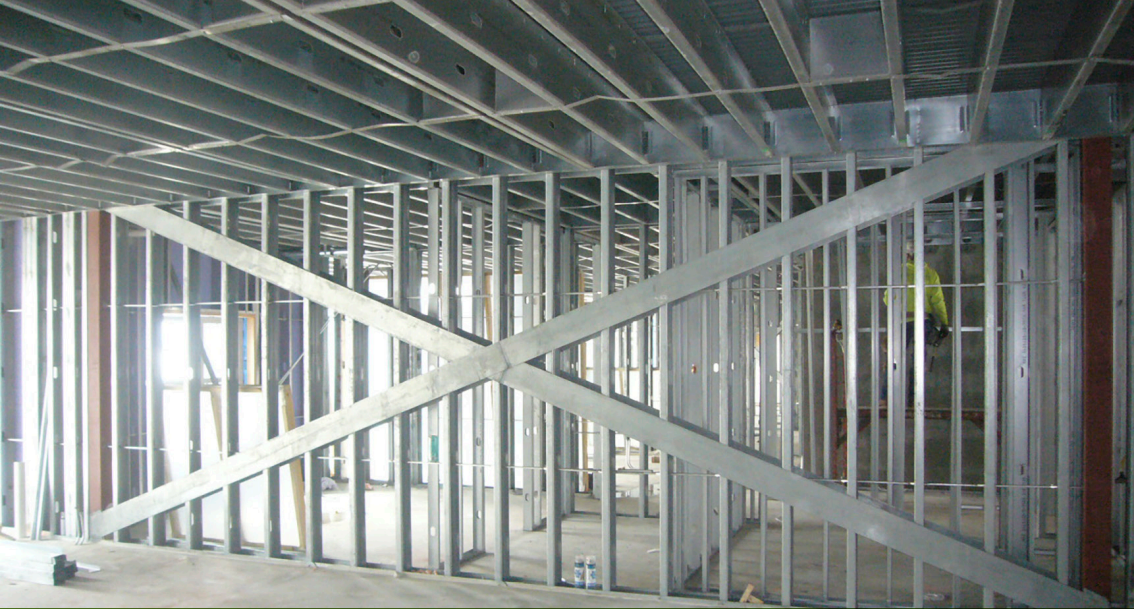
Metreau Apartments' lateral-resisting system includes X-braced CFS shear walls and pre-cast concrete stairs and elevator shafts.
