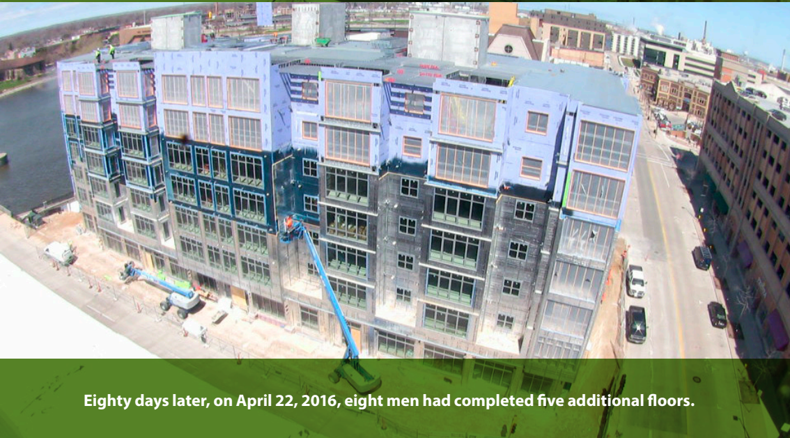
On February 1, 2016, erection of the CFS framing on the second floor of Metreau Apartments was nearly complete.
