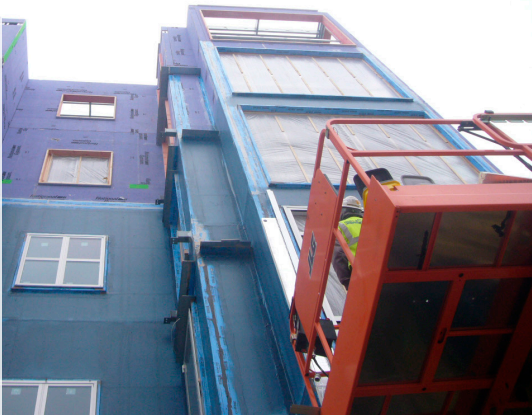
Metreau Apartments' framing design includes CFS attachment points for a variety of balcony types.
