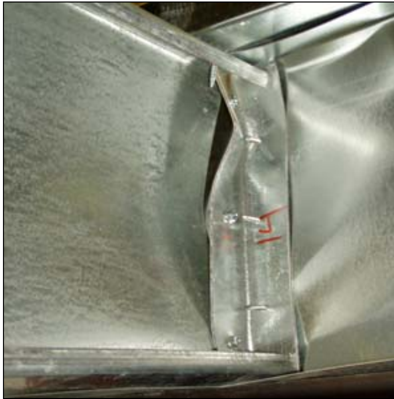
Figure 6.3 Screw Failure
