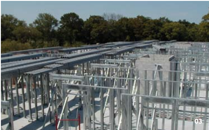
02 The steel for the wall studs and panels ranged from 1.9 mm (0.075") at the first floor to 1.22 mm (0.048") on the top floor. The steel floor deck is 1.52 mm (0.060"). By Jeff Wilkinson
