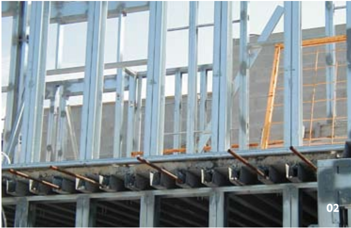
02 The steel for the wall studs and panels ranged from 1.9 mm (0.075") at the first floor to 1.22 mm (0.048") on the top floor. The steel floor deck is 1.52 mm (0.060"). By Jeff Wilkinson
