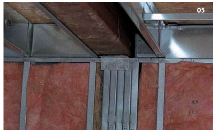
04 High quality cold-formed steel sections and panelized assemblies made from Dofasco Galvalume Plus and galvanized CFS are easily handled, economical, non-combustible and offer great design flexibility. 05 Genesis™ pre-engineered and pre-assembled panels were used to frame both the townhomes and the garages. 06 The roof truss system used for the garage roofs was assembled on the ground and then lifted up into position. 07 Heat transfer or thermal loss is not a problem for homes framed with pre-assembled panels made from CFS sections. Use of exterior rigid insulation mitigates heat transfer by thermal bridging. The wall assembly can be constructed to meet any required level of thermal resistance.
