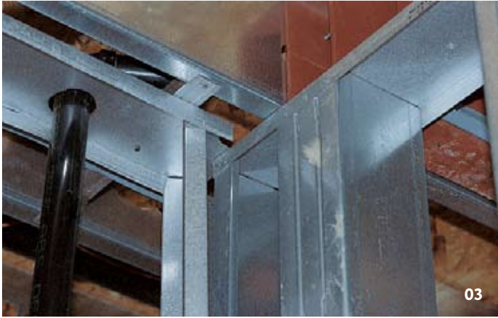
03 Steel framing is pre-punched for electrical wiring. Heating and ventilating ducts, plumbing and drain pipes can readily be installed.
