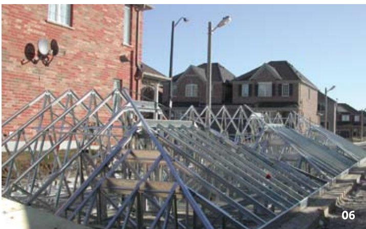
04 High quality cold-formed steel sections and panelized assemblies made from Dofasco Galvalume Plus and galvanized CFS are easily handled, economical, non-combustible and offer great design flexibility. 05 Genesis™ pre-engineered and pre-assembled panels were used to frame both the townhomes and the garages. 06 The roof truss system used for the garage roofs was assembled on the ground and then lifted up into position. 07 Heat transfer or thermal loss is not a problem for homes framed with pre-assembled panels made from CFS sections. Use of exterior rigid insulation mitigates heat transfer by thermal bridging. The wall assembly can be constructed to meet any required level of thermal resistance.
