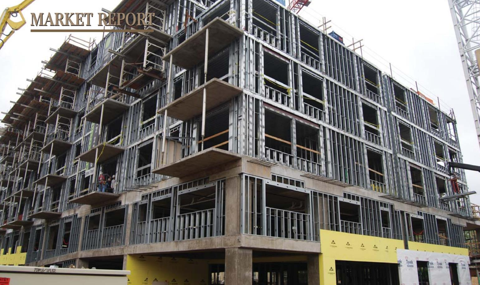
ble manner when subjected to the structural loads and stresses imposed by high wind or seismic forces. Steel studs cannot absorb moisture. This substantially eliminates the expansion and contraction of construction materials and the related cracks, pops, and other deformities in finishes.
