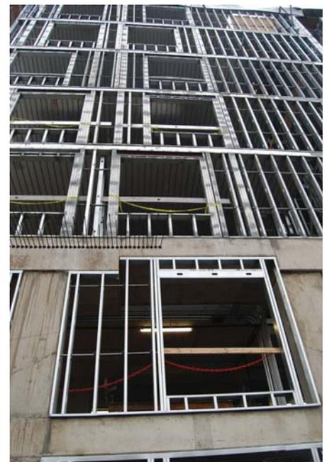
In the past, CFS has dominated the market for curtain walls and partitions in commercial construction, due to its light weight, high strength, non-combustible nature and ease of installation. But with advanced technological developments like panelized systems, the building community has started using CFS for structural applications on mid-rise buildings as high as nine stories.
