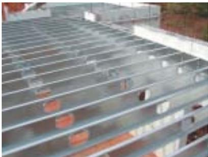
*Steel floor joists that are set after the concrete has been poured into the ICF.*
