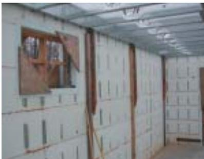
*Bracing is set just under the rim track to ensure it is level around the perimeter of the wall.*
