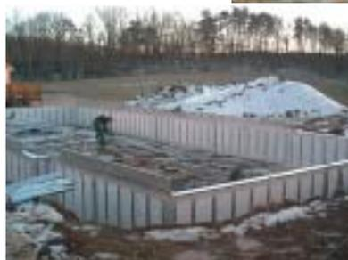
*Panelized steel systems, which are similar to structural insulated panels, are one alternative to concrete (far top).*
