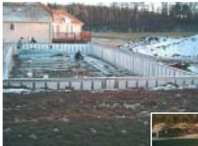
*The panels are either mechanically interlocked (with fasteners) or welded together. Whichever system is employed, the panels can be successfully used as basement or foundations walls.*
