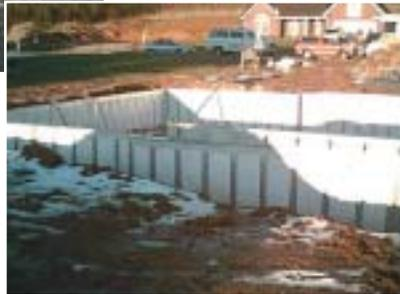
*These systems eliminate the need for a concrete contractor, as poured concrete walls are not needed and footings can be poured without a concrete contractor.*
