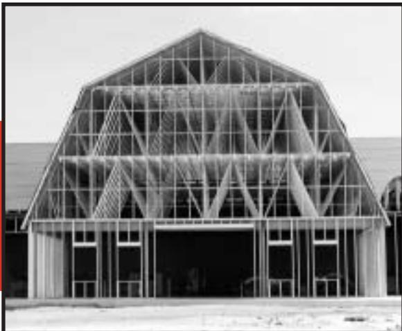
**A Rinker Materials/Bethlehem Steel joint venture, Steel-Con produces light-gauge steel roof and floor trusses, plus framing and accessories for walls and floors.**
