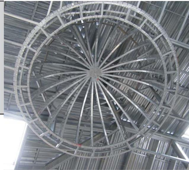
One of the things he likes best about building with steel is its design flexibility, and says it is easy to frame barrel ceilings, domes (pictured here) and other details with steel.
