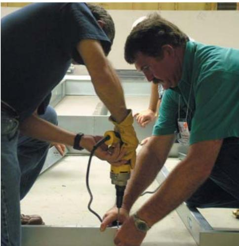
*During training, students learned the proper techniques for using tools in cold-formed steel framing. The student in this photo is using a screw gun designed for steel-to-steel connections.*
