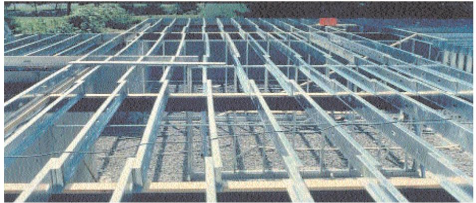
Figure B: Single span joists
