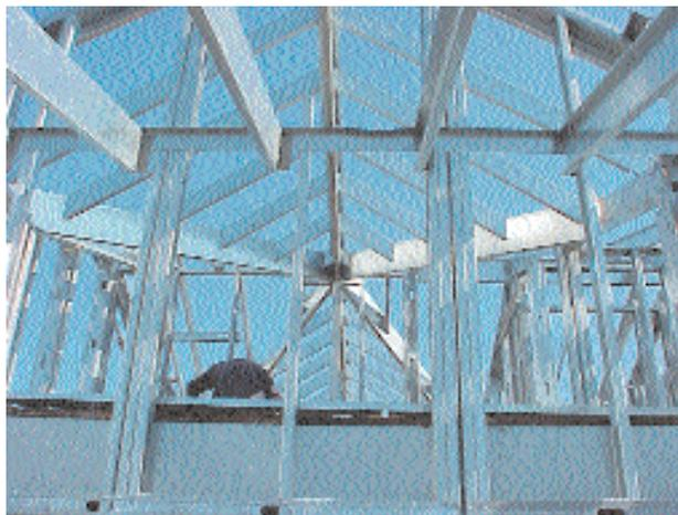
ing. Connections are sealed with adhesive, supported with brackets and welded.
