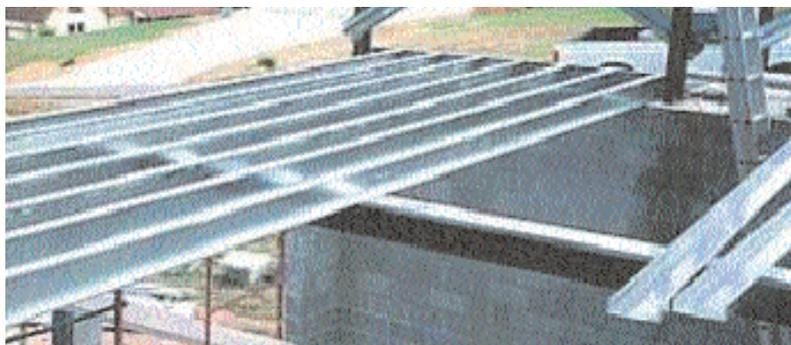
Figure A: Continuous joists
